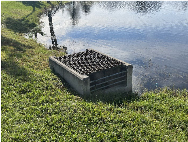
P-13C Control Structure
