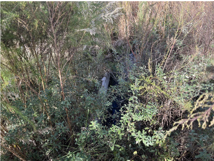
P-2 Outfall MES- removal of overgrown debris/vegetation.
