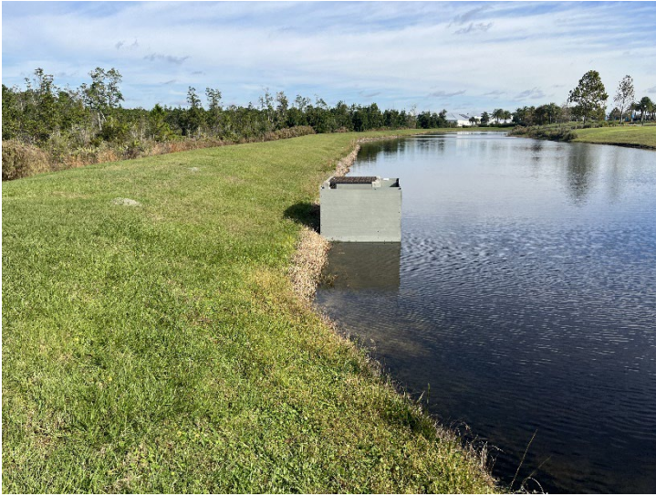
P-2 Control Structure
