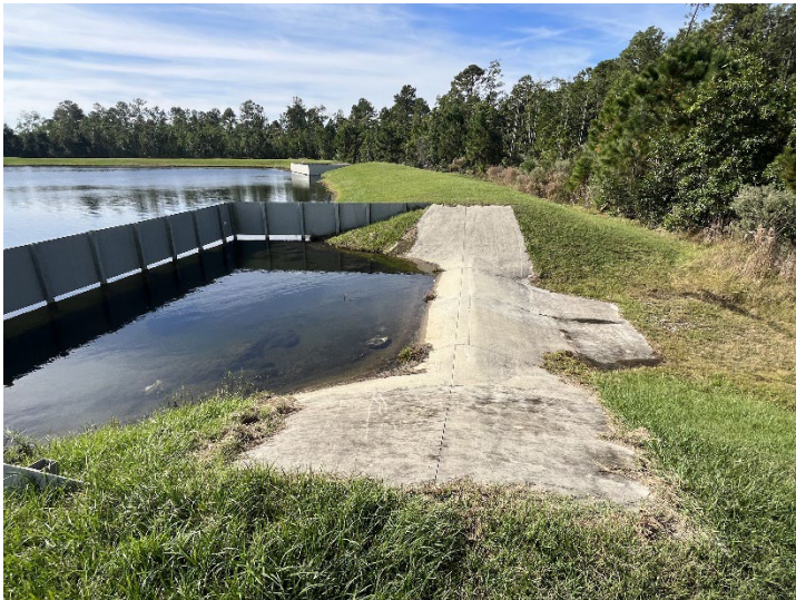
P-1 Outfall Spillway #1
