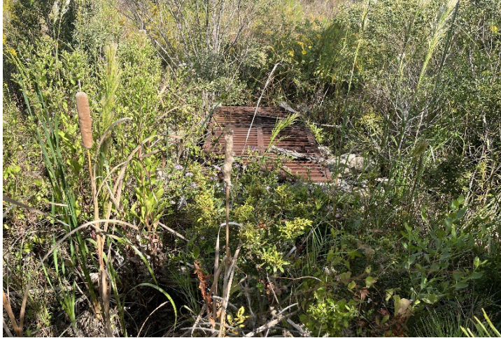
P-14D Entrance Culvert
