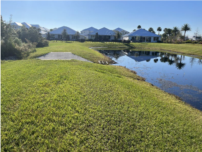
P-15C, View Facing West Spillway Structure clear of Debris.
